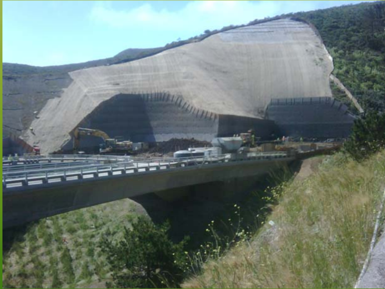
Jute Mesh Matting w/ Wattle Check Dams →
