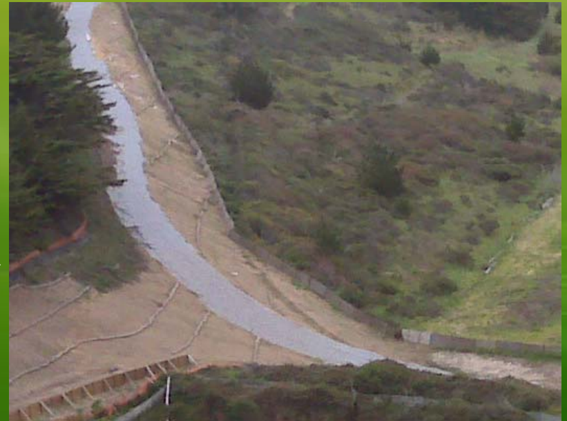
Jute Mesh Matting w/ Wattle Check Dams →
