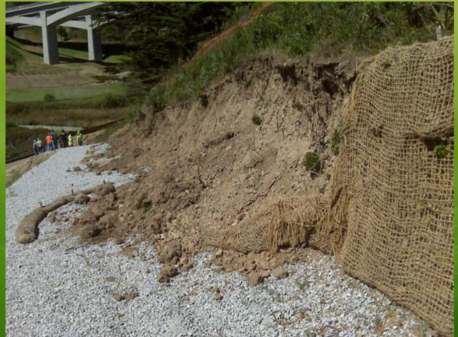
Hillside blowout on access road
