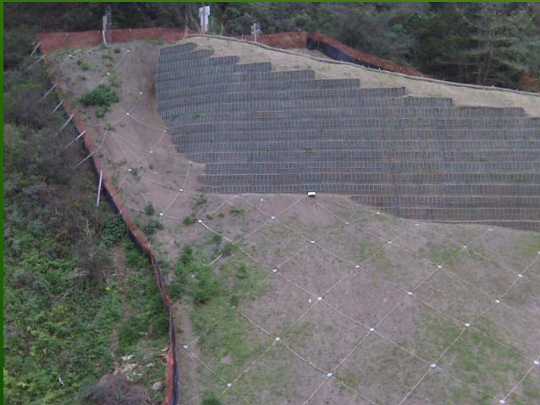
← Reinforced Jute Mesh Matting
